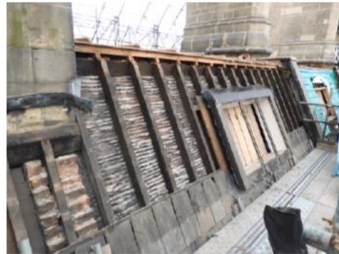
5.109 Slate and battens removed from roof slope WR18 Thursday 16 June 2022
