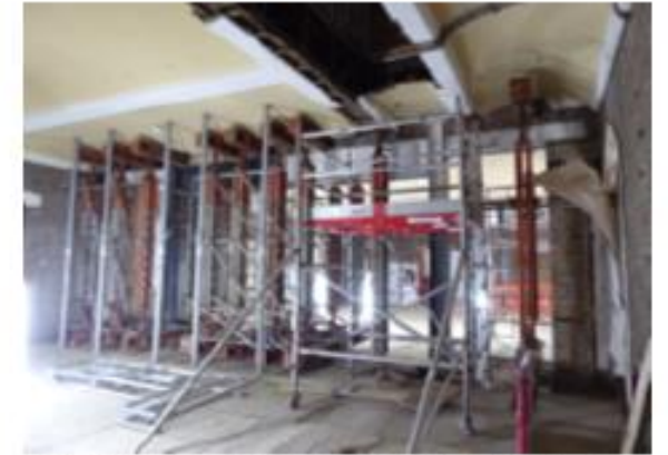
5.12 New opening on the east side of room 04-024 Tuesday 15 March 2022
