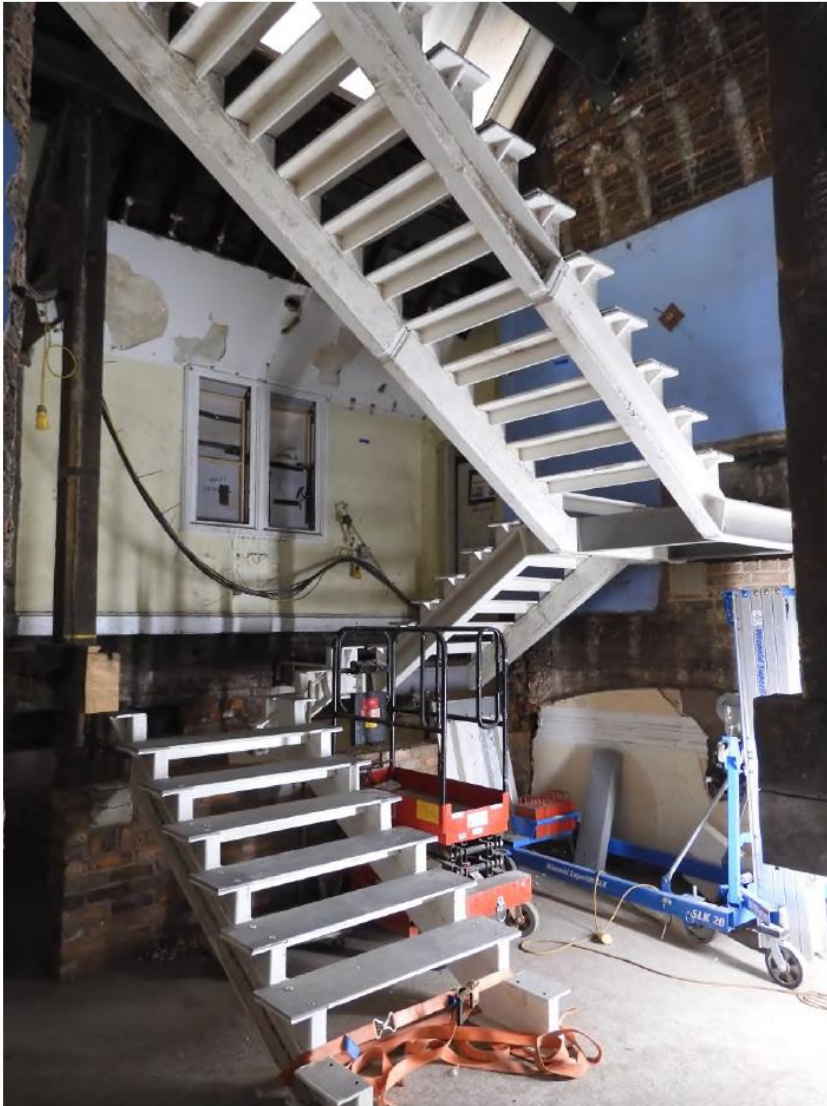
5.8 New stair S20 at level 5 Tuesday 26 July 2022
