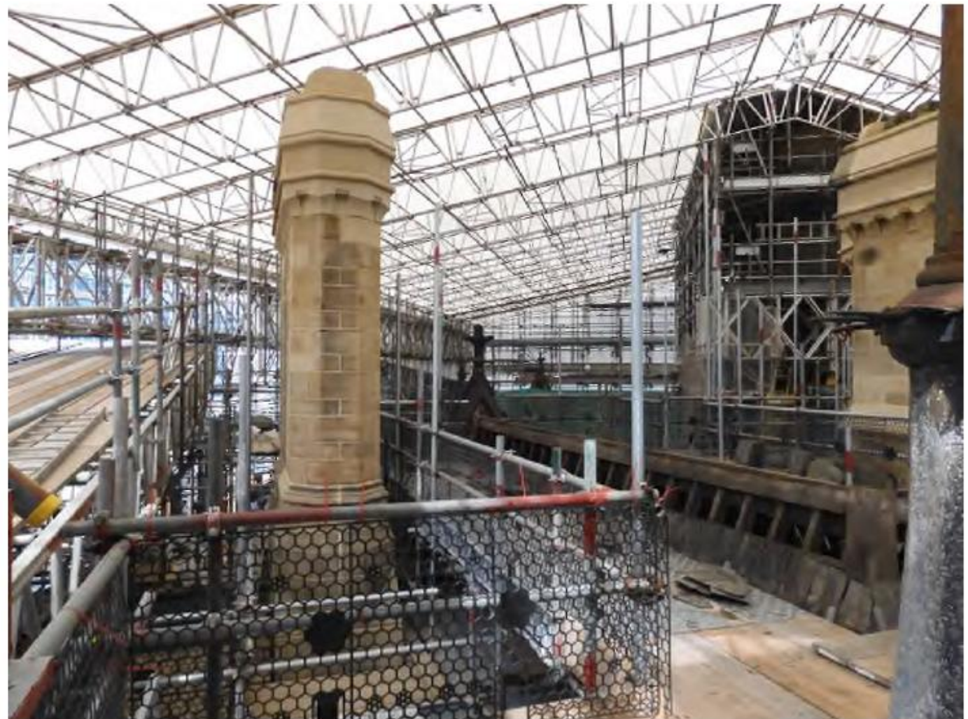
5.2 Cooper Street temporary roof viewed from inside from south to north
