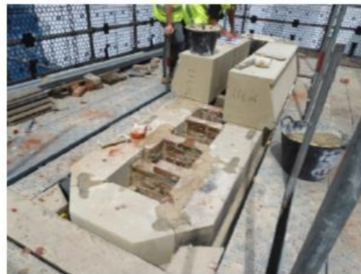
5.89 Top of chimney CS21 viewed from south Tuesday 7 June 2022
