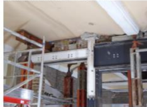
5.13 Brick infill installed above steel beams to opening in room 04-024
