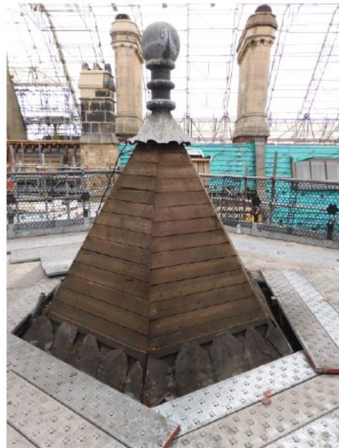
5.112 Slate and battens removed from top of roof WCR10 Thursday 16 June 2022
