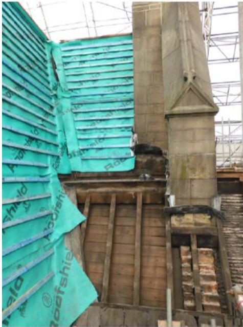
5.110 Roof slopes WR19e Thursday 16 June 2022
