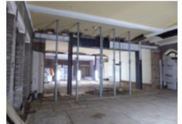
5.16 Overview of room 04-024 from south-east corner
