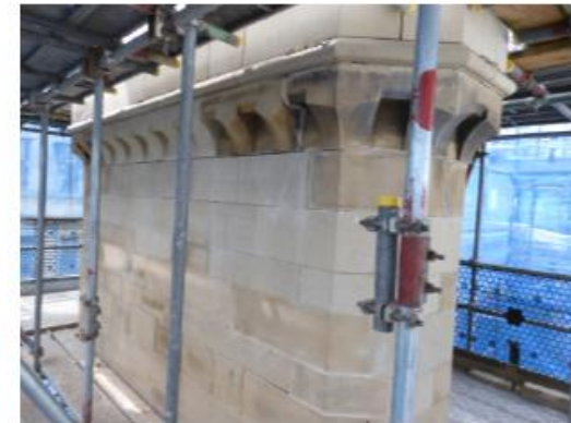
5.87 Chimney CS21 viewed from south-west Tuesday 7 June 2022
