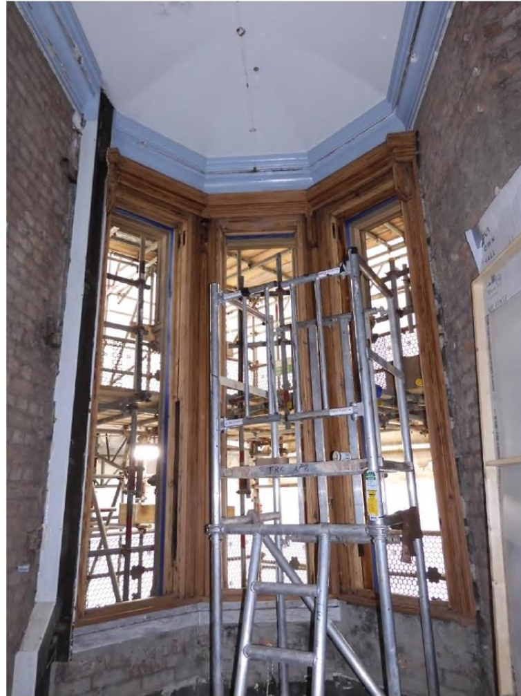
5.40 Preparation for painting sash window frames underway in room 01-019
