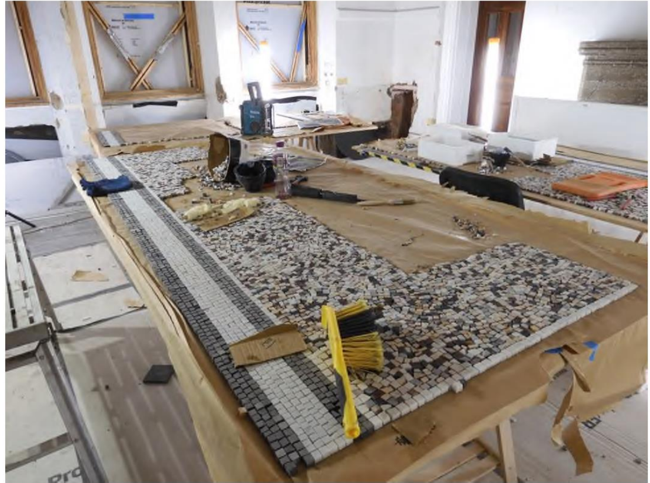
5.36 Preparation of mosaic panel underway in workshop on level 1
