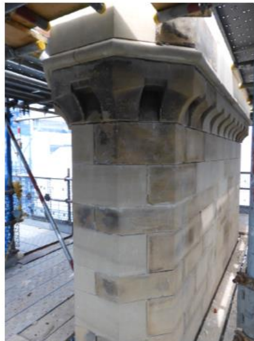
5.88 Chimney CS21 viewed from south-east Tuesday 7 June 2022
